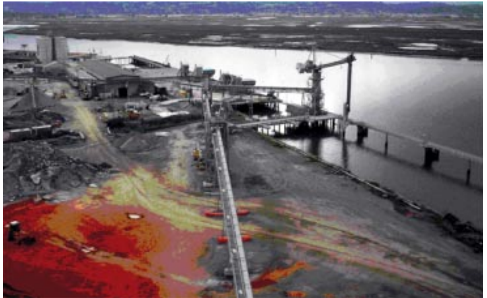
Warehouse 1 and Wharves 1 & 2
