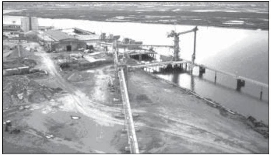
Warehouse 1 and Wharves 1 & 2
